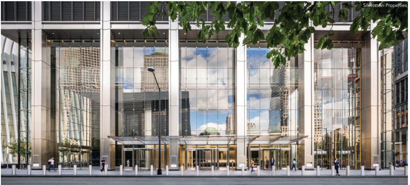
The high-strength duplex stainless steel S32205 mullions in the glazed façade of the 60-ft-tall three-sided atrium to 3 World Trade Center are sharp-cornered profiles of built-up structural tube, which was selected for its resilient design characteristics and excellent corrosion resistance.
